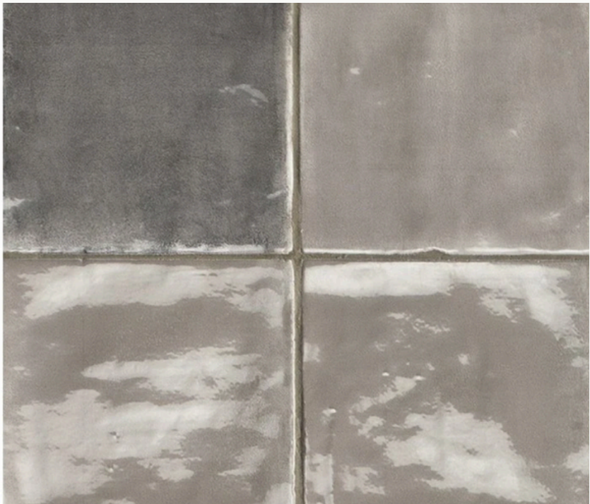
SHOWER WALLS & BENCH
